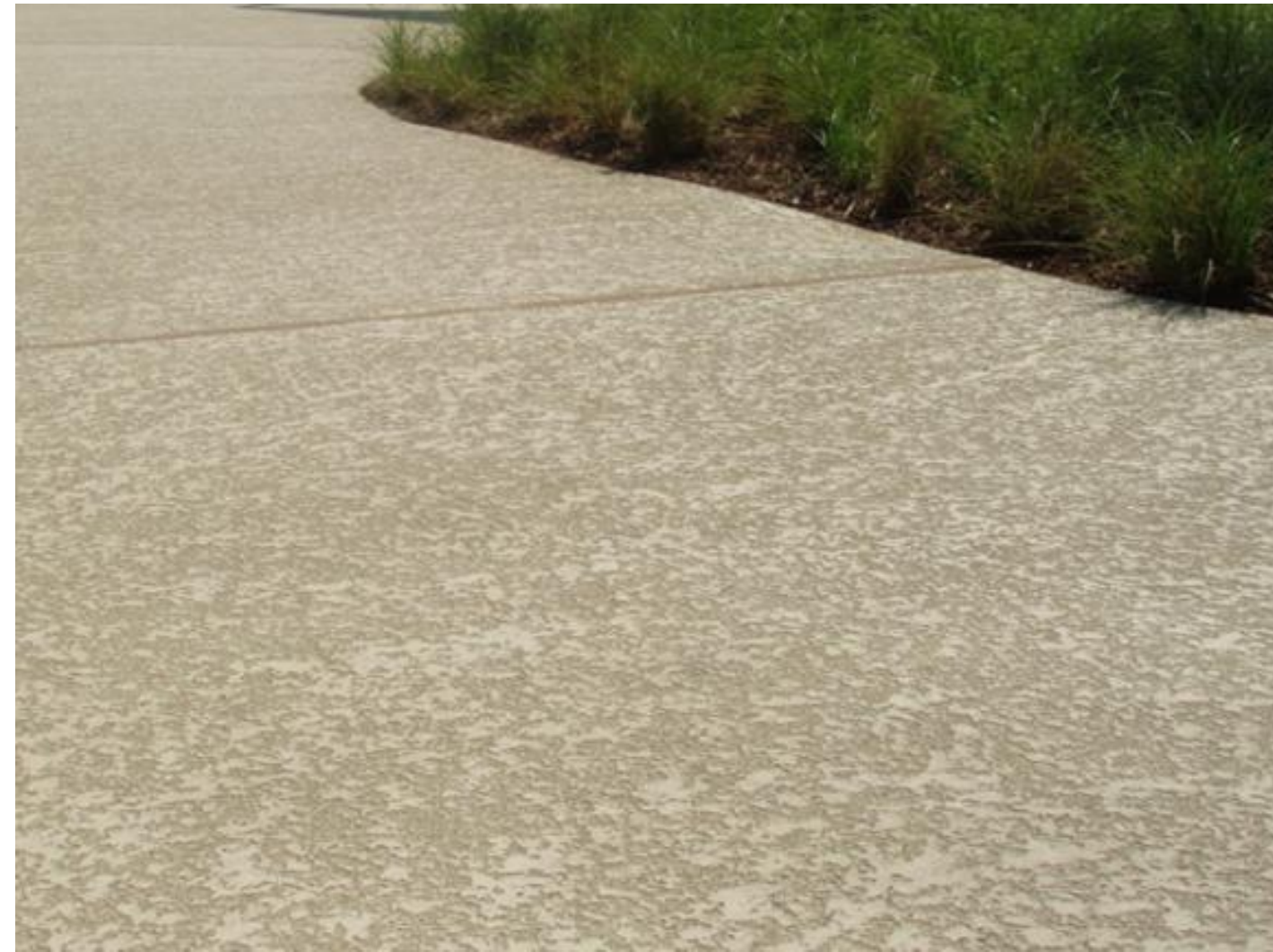
SPRAY DECK FINISH TO CONCRETE
